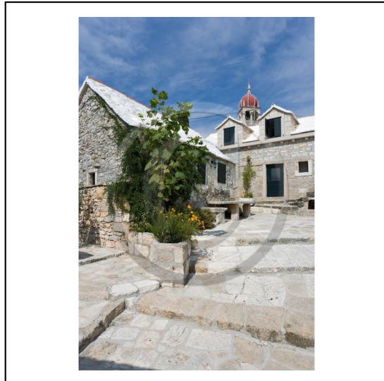
Croatie, Ile de Brac, Donji Humac, Maison traditionnelle restaurée, toit de pierre // Croatia, Island of Brac, Donji Humac, traditional house restored, roof of stone
